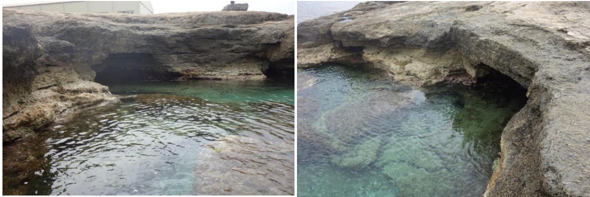
Fig. 39 – Rock cutting on the north of the current slipway
