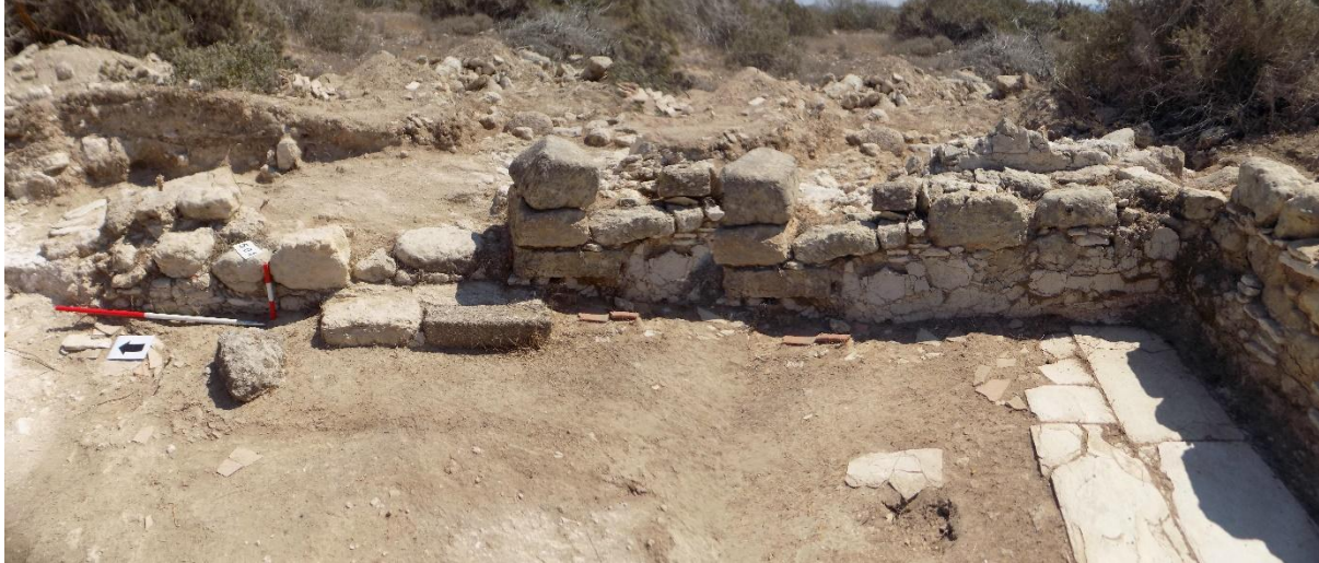
Figure 24: The south-east corner of the hill-top structure.
